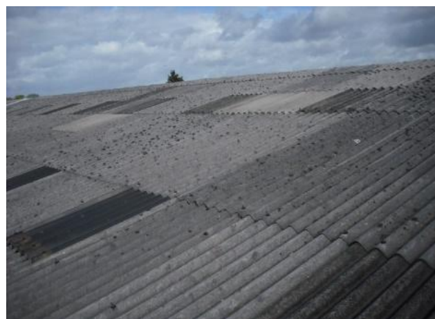
Fig. 2 Coverings from asbestos cement
