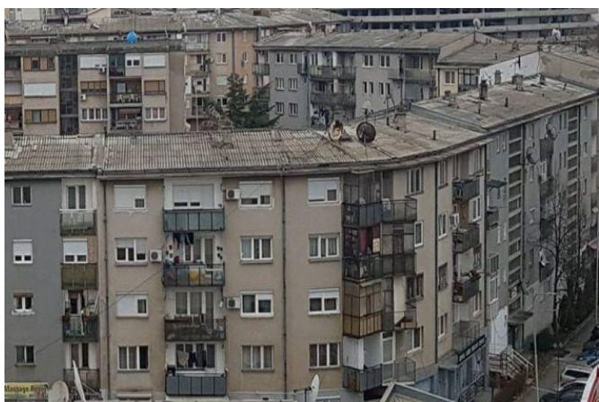
Fig. 1 Buildings in Pristina covered with asbestos cement
